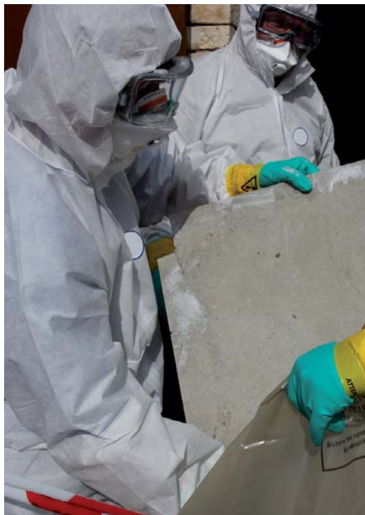
Handling of asbestos boards.
